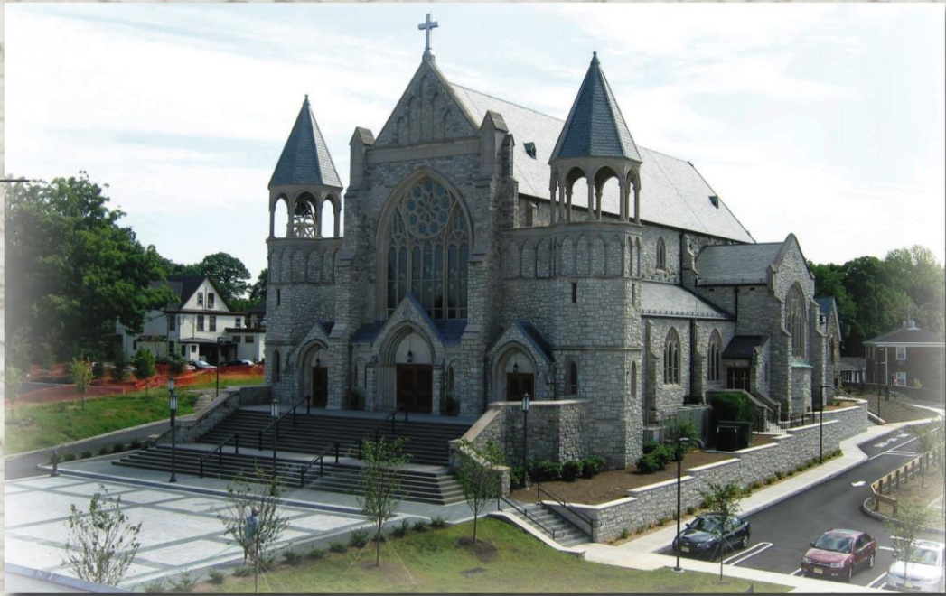
St. Teresa's of Avila in Summit, NJ. Complete interior renovation and exterior restoration of the site and grand plaza area.
